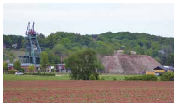
Fig. 7. The Röhrigschacht mine near Wettelrode is open to visitors as a museum and show mine today (photo: A. Swieder).
